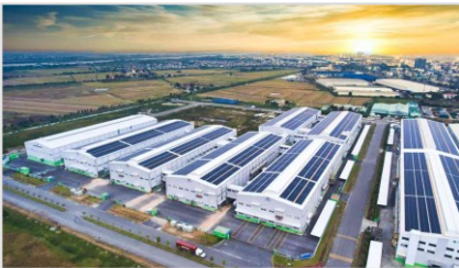
Figure 4.5: Rooftop solar installation (Source: SkyX Solar)
