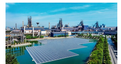
Figure 2.13: Solar power at the regulating lake, over 2,500 kWp, phase 2 completed in June 2026 (Source: Hoa Phat’s website)
